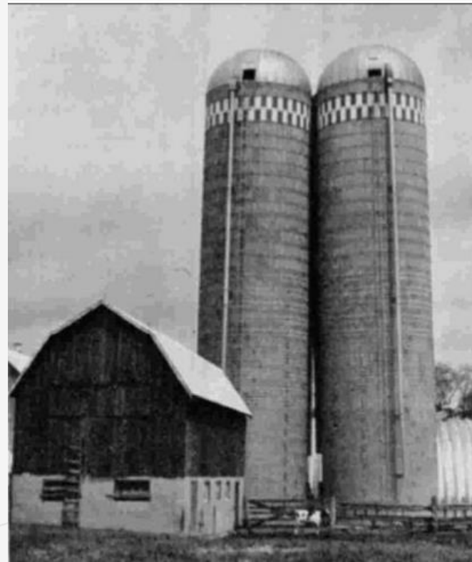
Tilting adjacent silos
